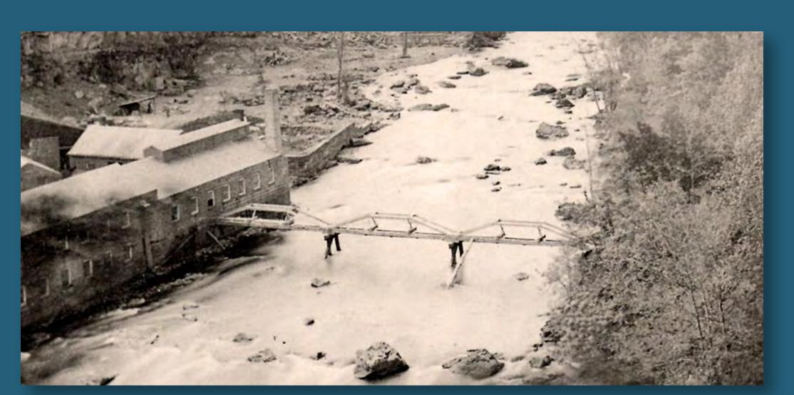
The Passaic Water Company's first pump house of the 1850s was in a complex of mills below the Great Falls, later redeveloped as the Allied Textile Printers (ATP) Site. Water was pumped across the "broomstick" bridge, shown here in a photograph of about 1870. The bridge's pipe sent water to a reservoir in the area of Hinchliffe Stadium, directly behind you. Image Credit: Paterson Historic Preservation Commission.
