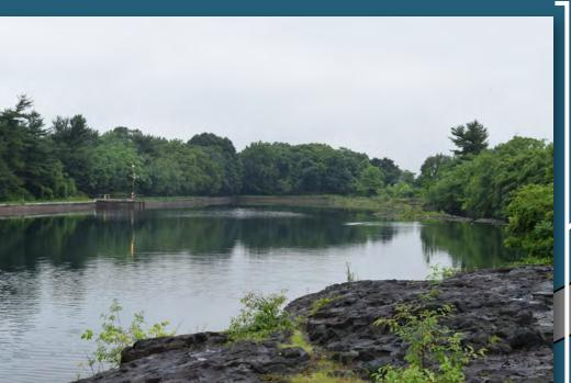
The reservoir's outlet chamber pulled water from the reservoir for disinfection and distribution to customers. This outlet chamber and old chlorine station was constructed of concrete in 1932-33, replacing an earlier stone chamber.
