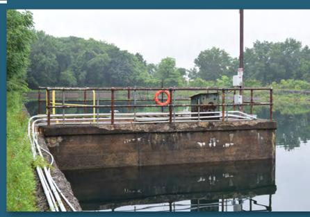
The reservoir's inlet chamber drew water from the Passaic River to fill the reservoir. The chamber was constructed of reinforced concrete and added in 1932-33.
