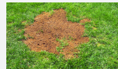
Temporary backfilled holes in your yard are filled with soil and left to settle.
