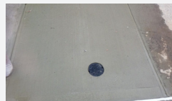
Permanent sidewalk repair at the curb stop.
